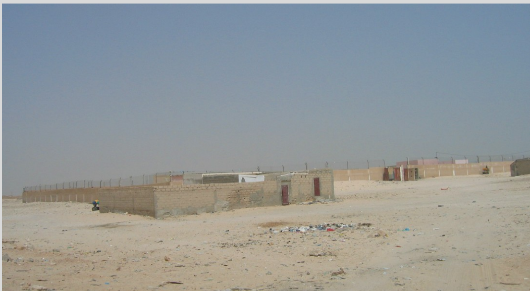
© AI – Nouadhibou Detention Centre
